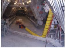
The blower is located away from the work area. The inflation tube can be furnished in any length required. If two blowers are required to meet redundancy requirements, a "Y type inflation tube can be supplied as two blowers can be connected at the same time.
