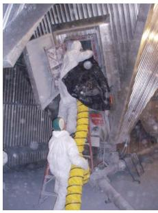
The duct balloon easily passes through the existing 27" x 21" man way during installation and weighs less 25 lbs. Installation time takes minutes, not hours versus scaffolding.
