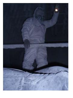
The platform inflates in less than one minute and can support the weight of two people. For this application, the inflatable serves as a temporary platform so that pick boards can be loaded into the precipitator. The pick boards will provide a rigid platform so that maintenance can be safely performed on the electrical components.
